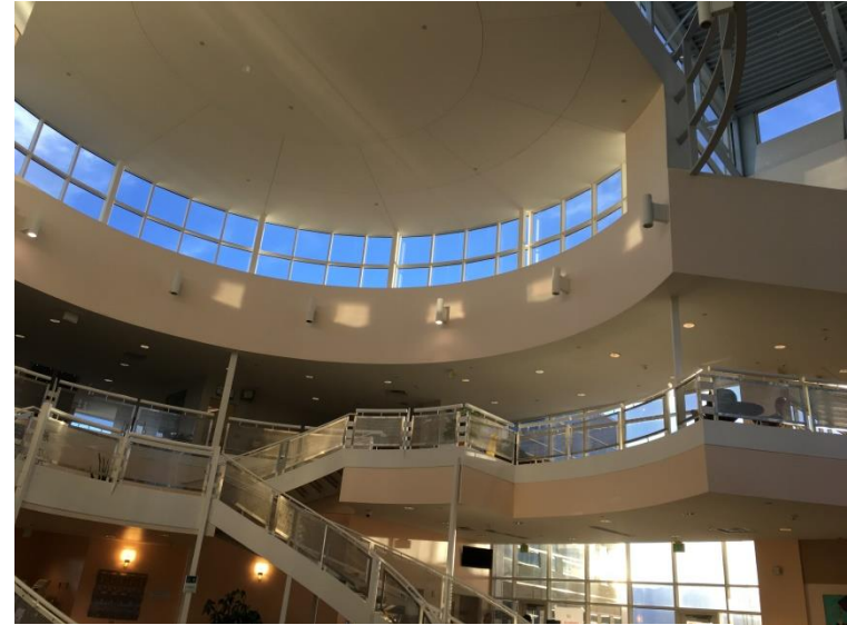
View in the atrium space
