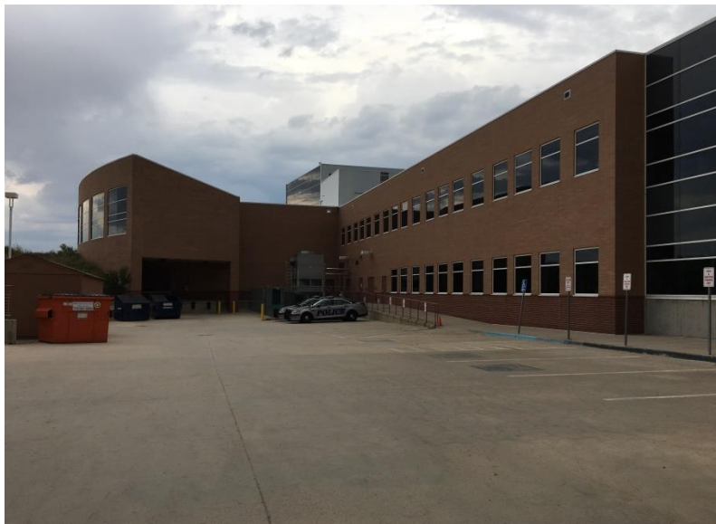
Figure I. Rampart Range Campus, west side view of the North Wing at the loading dock.
