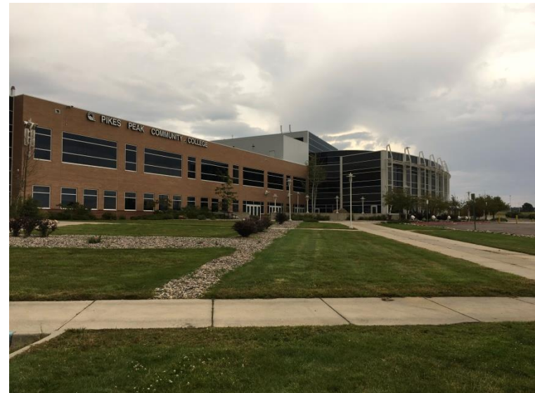
Southwest view of the Rampart Range Campus main building
