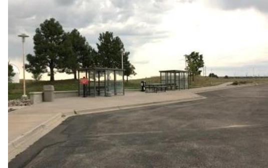
Figure B. Bus stop.
