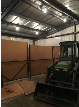
Existing engineered building, possibly repurpose into indoor Candidate Physical Abilities Test (CPAT) space.
